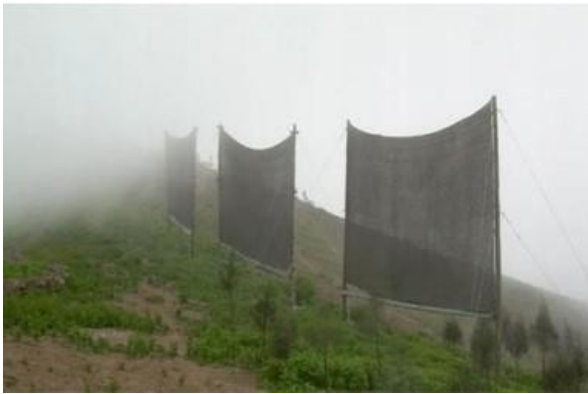
Photo 7. Water harvesting nets in the Chilean village of El Tofo. www.nicolabarbisan.files.wordpress.com .
