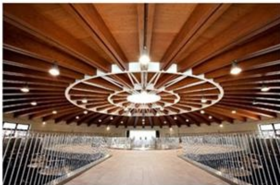
Photo 2. Antinori "la Mortelle" winery in Tuscany. It was designed to limit the impact on the environment with optimal integration into the surrounding hills. The cellar has a semi-buried hemispherical shape, hidden for the most part in a hillside and vegetation in the unburied areas. A skylight provides natural lighting inside the cellar. Photos www.antinori.it .
