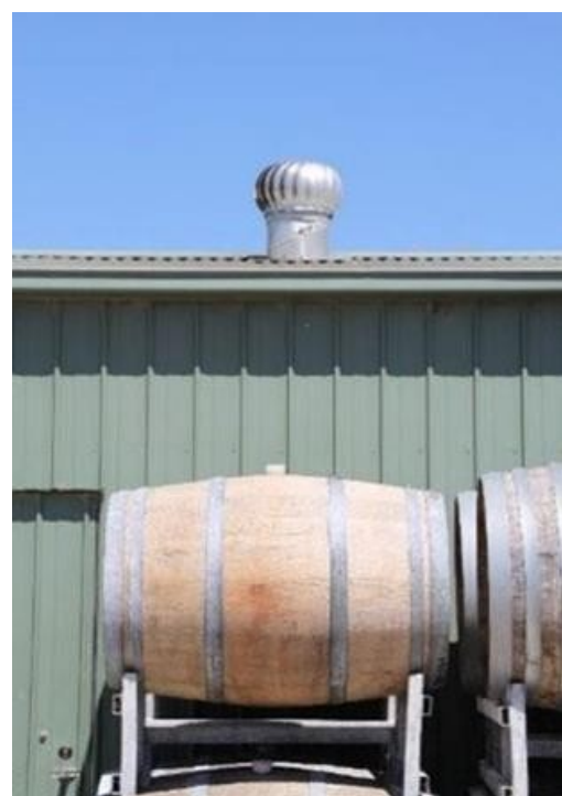
Photo 7. Example of under-roof warm air extraction in the McLaren Vale region of Australia, photo J. Rochard.
