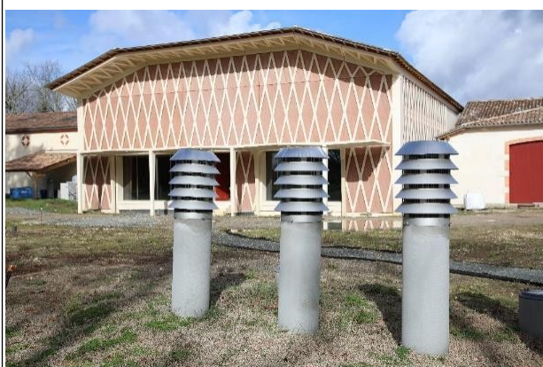
Figure 22. Example of a Canadian well at Château de Malleret in the Médoc, photos J. Rochard.
