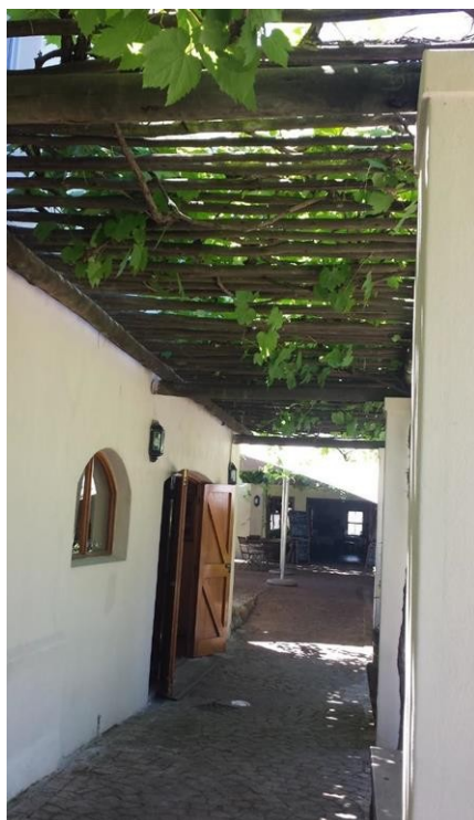
Photo 4. Vineyard pergola near the administrative buildings, which filters light in the summer and retains natural light in the winter, Photo J. Rochard.
