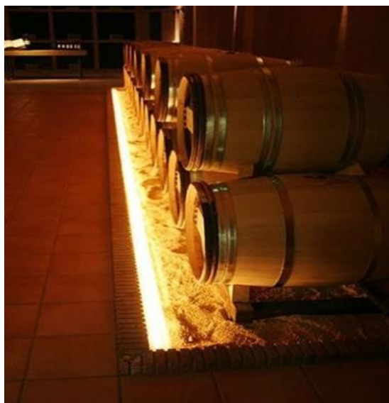
Photo 8. Natural humidity control in the cellar by maintaining the link with the subsoil in the barrel storage area. Photos J. Rochard.
