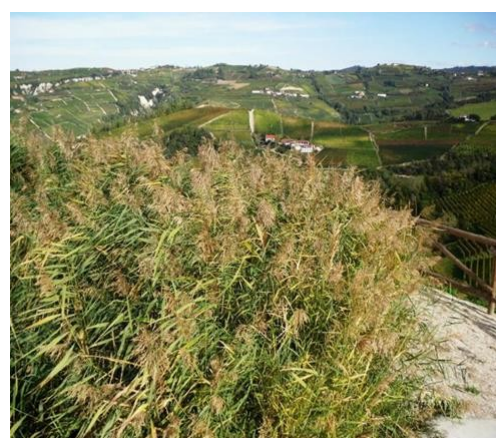
Photo 13. Effluent treatment using a reed bed on a zeolite support with the Zeofito® device (Baroli winery in the Italian Piedmont). The treatment system, which does not cause any nuisance, is installed directly in the visitor circuit, near the winery.
