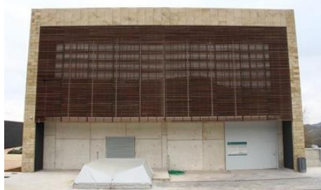
Photo 5. Sun breaker" device at La Grajera, a Gobierno winery in the Rioja region of Spain, photo J. Rochard.
